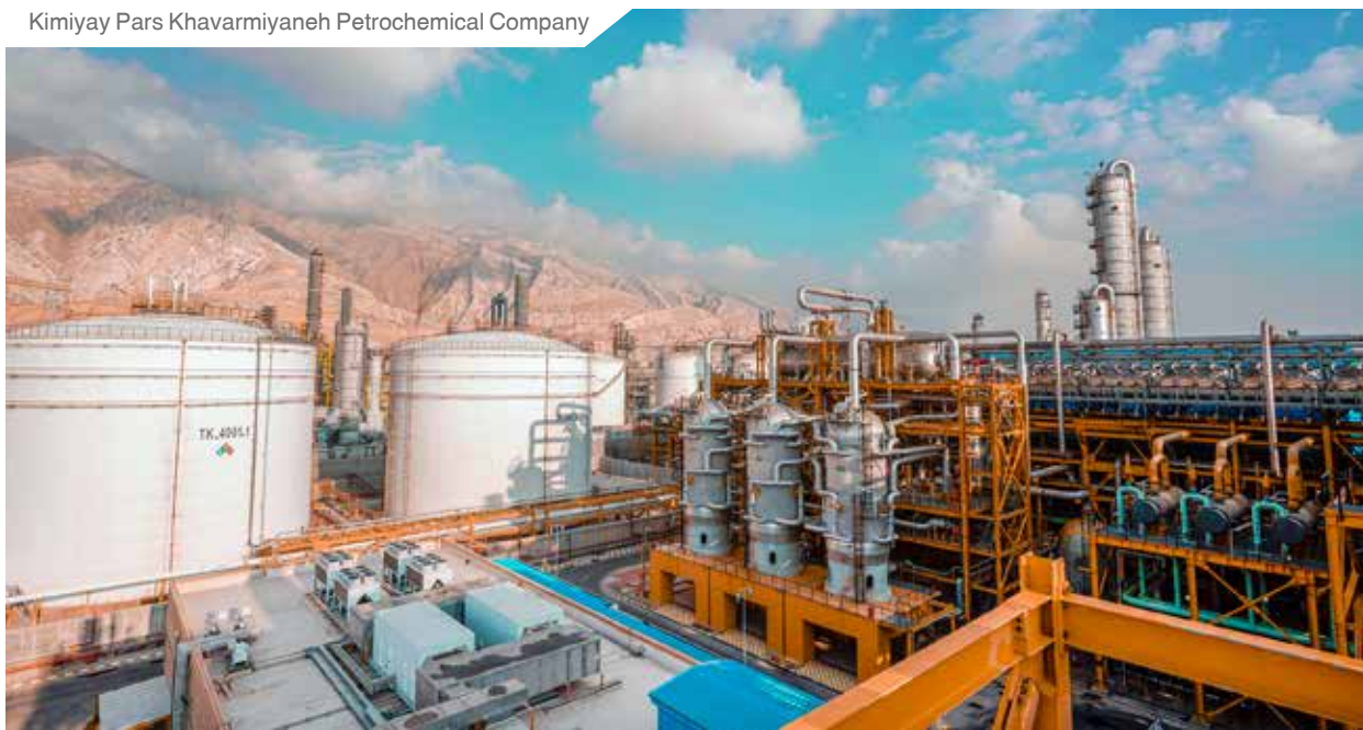
Kimiya Pars Khavarmiyaneh Petrochemical Company
